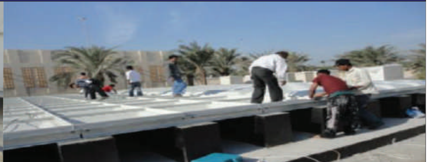
Installation of New Tank
