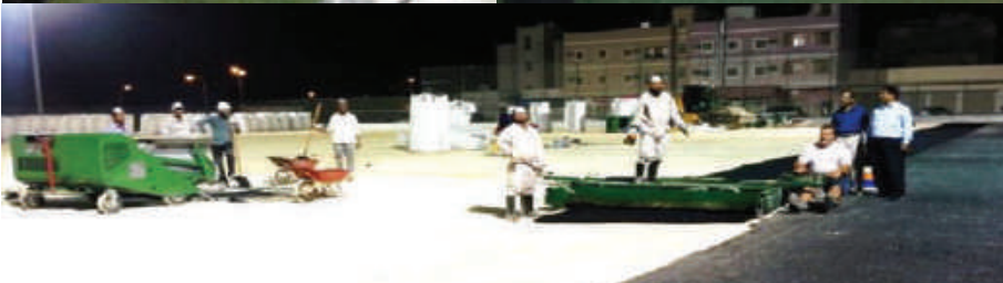
Mr.Pradeep Conducting site Inspection for Shock pad Preparation (Underneath of Foot Ball Turf ) World Class
